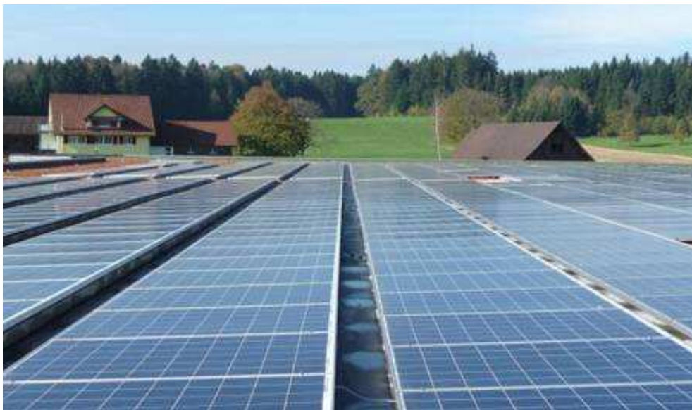
Partial view of the flat roof of the new goods depot. The horizontal arrangement of the solar modules makes good use of the roof's surface area.
