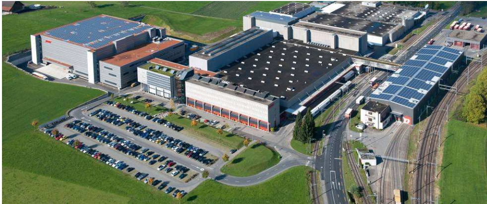
View of the Pistor AG office and warehouse complex with solar power facility.
