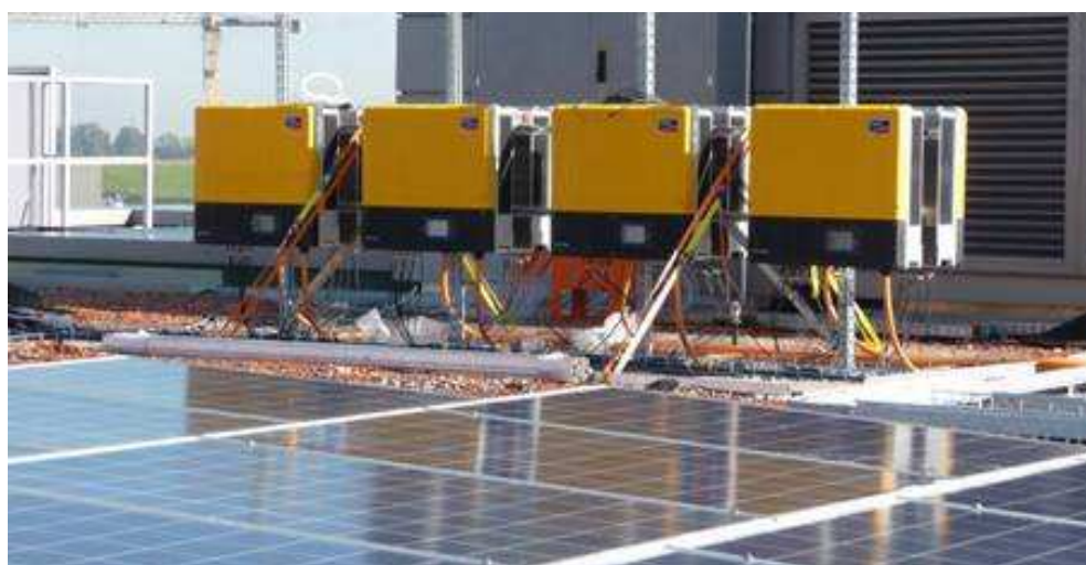
The newest generation of inverter attains the highest level of efficiency, some 98%.
